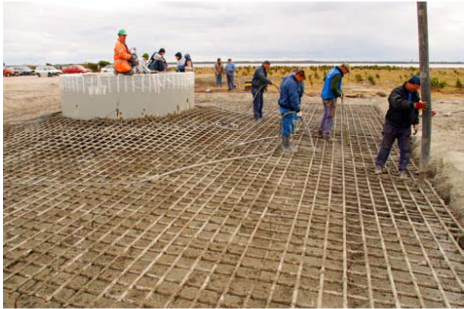
Gravitationsfundament. Foto: Gunnar Britse, WindPower Photo.
